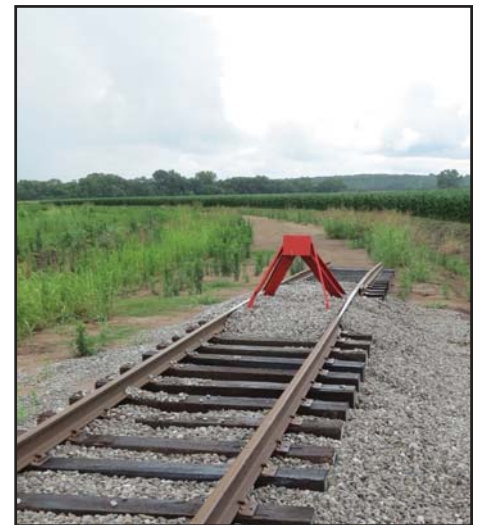
What used to be the end of the Union Pacific rail line is now the beginning of International trade opportunities at Iron Horse Industrial Park in Oklahoma
