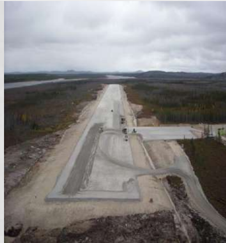
Airstrip construction Credit: Agregat RN – Goldcorp's Eleonore mine
