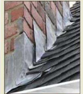
Lead chimney flashing
